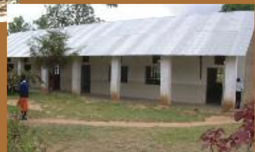
Malindi Suji Secondary School refurbishment.
