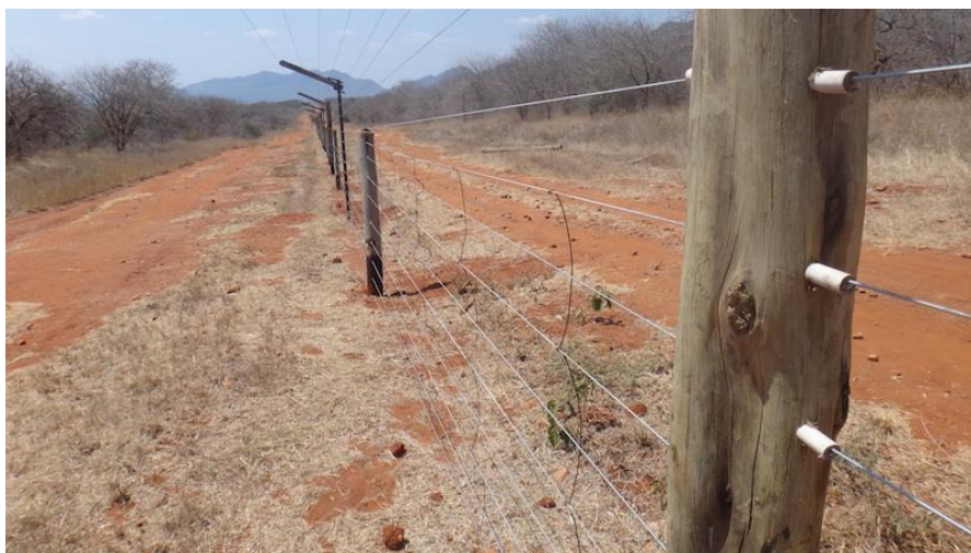
The new fencing configuration; droppers and rings on the lower half of the fence creating a broad and solid mesh
